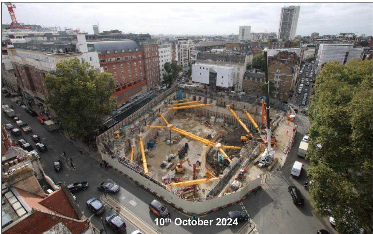
Above – progress in early October. The site has reached its full depth, and the bottom is flat and level.
